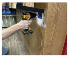
5 With a 1/4" drill bit, drill out the holes holes that had the screws removed.
